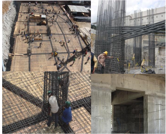
Fig. 7: Views of different stages of construction.
