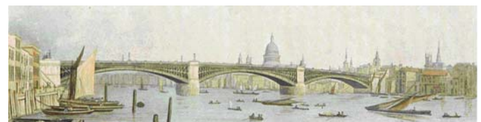
Fig.2 Southwark Bridge, London, 1819: Iron in the structural form of stone. The arches of the first iron bridges built approximately 200 years ago were constructed using traditional stone construction methods. In this case, curved iron blocks were used instead of stone, a technique that was used up until the development of the first steel frames.
