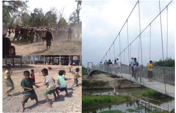
Fig. 1. Pedestrian bridge built from Toni Rüttimann (Toni "El Suizo"). Driven by humanitarian motivation, Toni helps people in need around the world to build wonderful cable supported bridges. Up to date nearly 400 bridges with up to 270m span have been built in rural areas at very low costs using cables, tubes and plates spent from the oil and steel industry. With his noble actions the bridge builder movement led by Tony has repeatedly demonstrated that a few simple engineering techniques combined with a precise bridge management system are key ingredients to make a better world.
