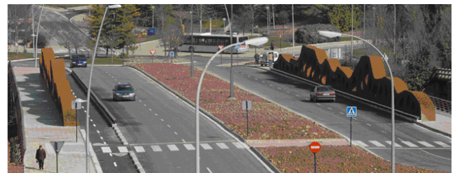
Fig. 3: Abetxuko Bridge over Zadorra River, Vitoria, Spain. This exceptional bridge has been designed by Dr.-Ing. Juan Sobrino.
