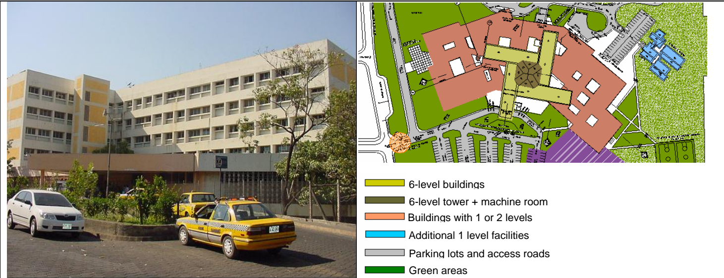
Fig. 3: Hospital de San Juan de Dios, located in San Miguel, El Salvador. This health care facility is amongst largest of its kind in Central America. It consists of four buildings of six levels each, and a series of 1-2 level buildings. Total constructed area is 37'126 square meters. Left: Front view. Right: Top view w. indications of the main areas.
