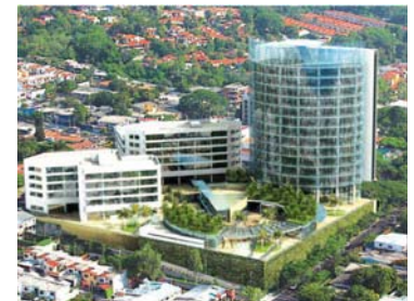
Fig. 4: Overview of the WTC III expansion project, including Torre Futura and adjacent buildings.
