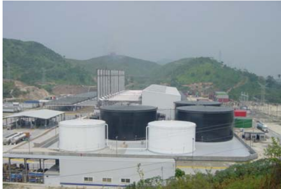
Fig. 6: Choloma III Diesel Power Plant, Honduras. Configuration: 15 X 18.6-MW 18V48/60 MAN B&W engines Fuel: heavy Oil Operation: 2004/2005.
